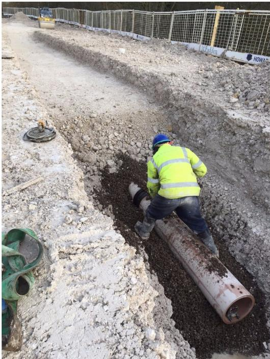
During the past 2 weeks we have been placing stone fill adjacent to the A19 in preparation for the piling works that will recommence after Christmas. We have also been installing drainage to the east of Fordlands Road.
